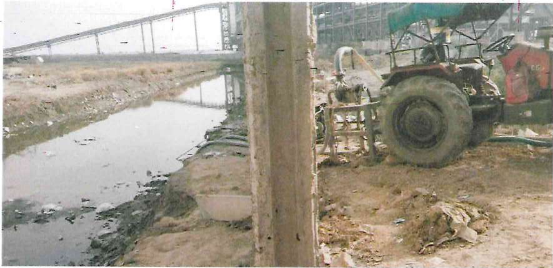
[Dewatering from the trench of Plot No.540]
