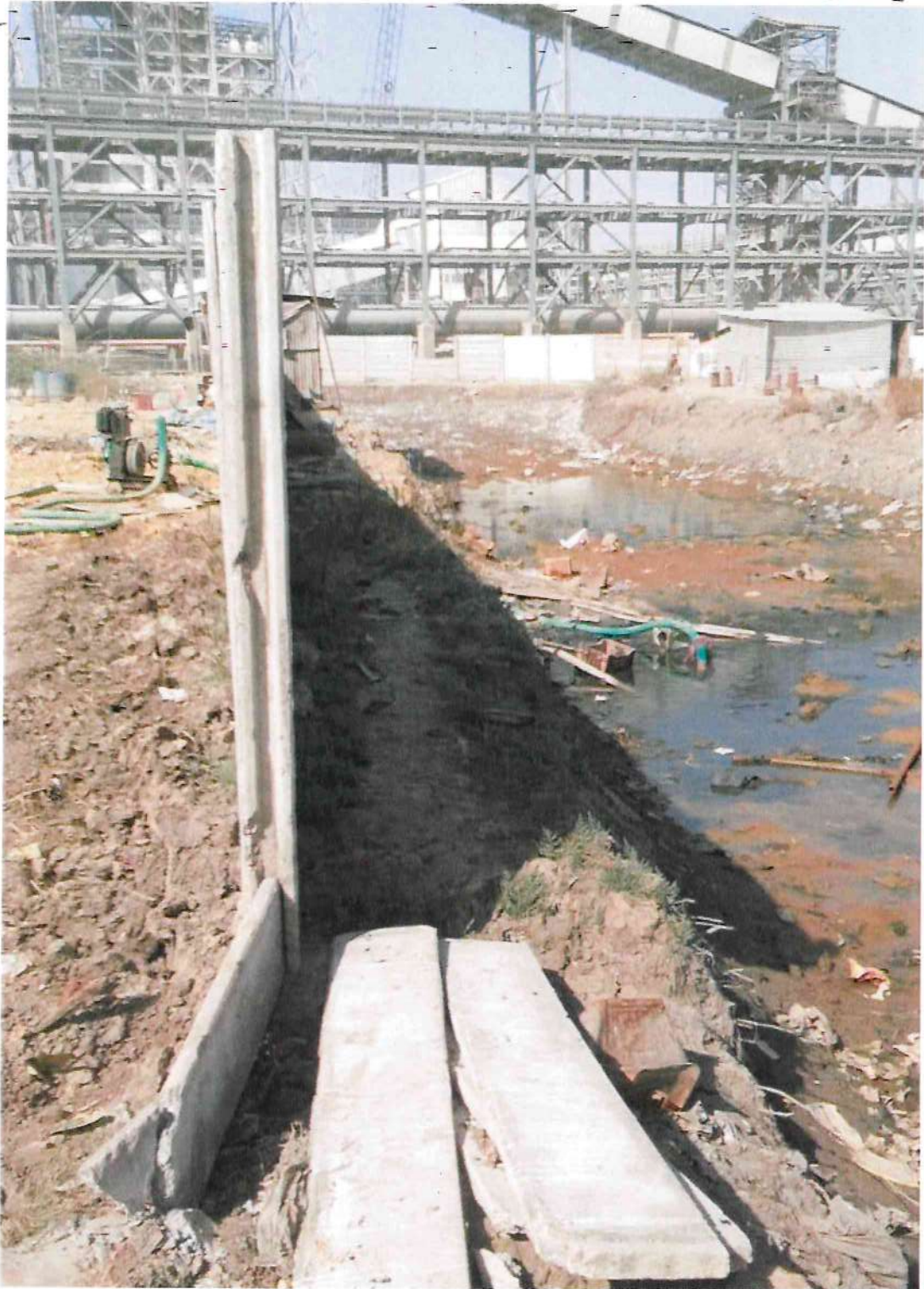
Dewatering activity from the plot of survey No. 540:
