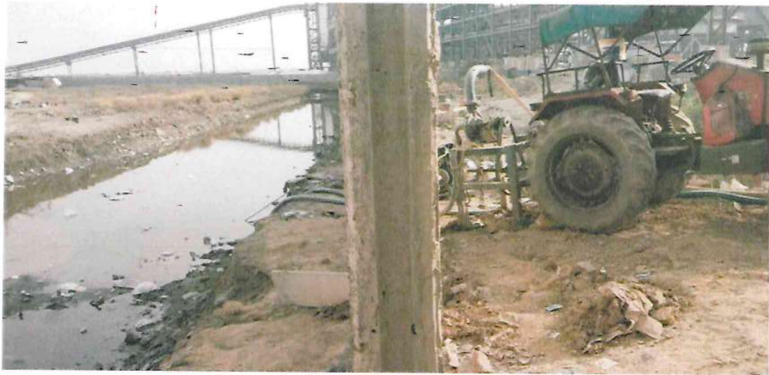
[Dewatering from the trench of Plot No.540]
