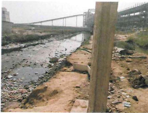
[After dewatering from the trench]
