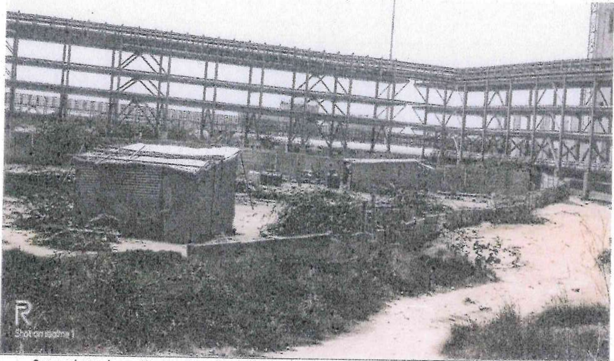
Some shops (unauthorized) are being operated in Survey No. 540/p-1 for commercial purpose
