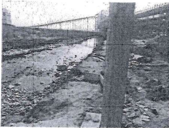
[After dewatering from the trench]
