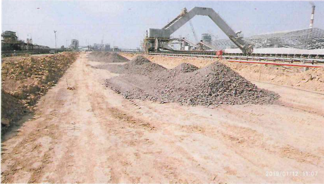
Photograph showing the progress of pukka road development:
