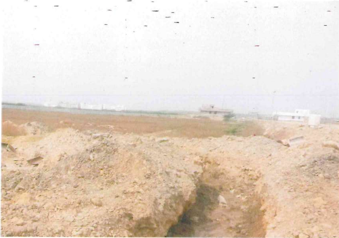
[Area near Plot No. 606 is dewatered]
