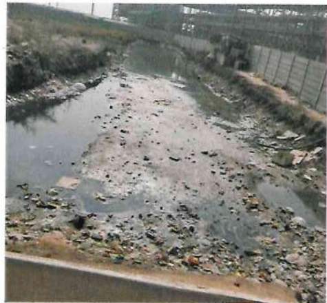
[Shop nr. trench and solid waste in trench]
