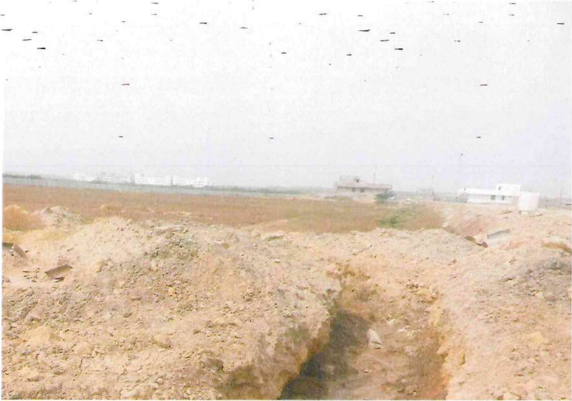
[Area near Plot No. 606 is dewatered]
