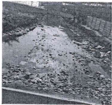
[Shop nr. trench and solid waste in trench]
